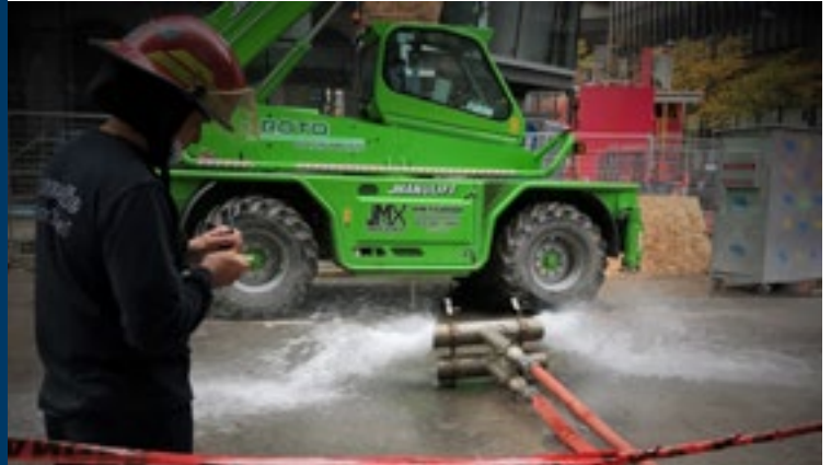
Supervising a flow test
