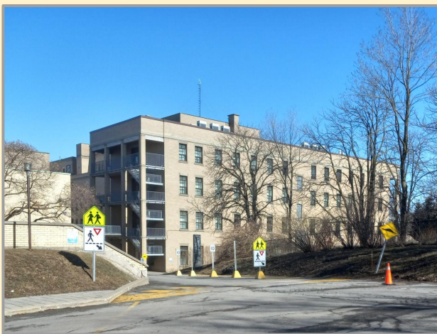
Centre Vimont (pavillon D), photo 2022.
