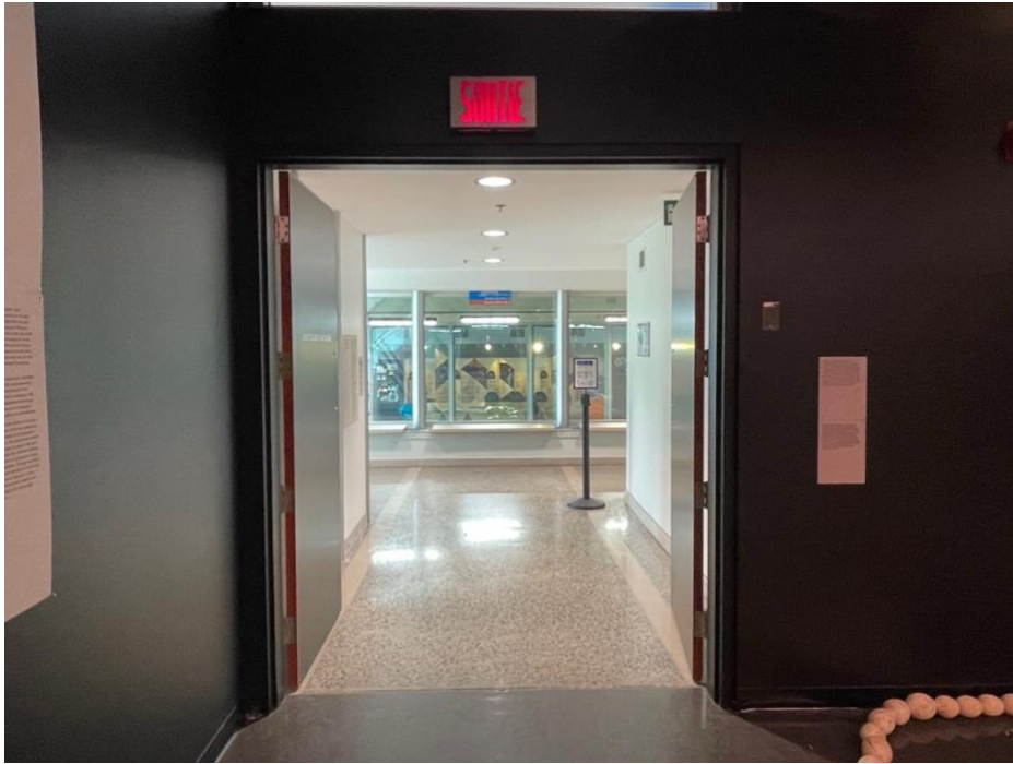
Room 4 public exit door - 172 (L) cm x 221 (H) cm
