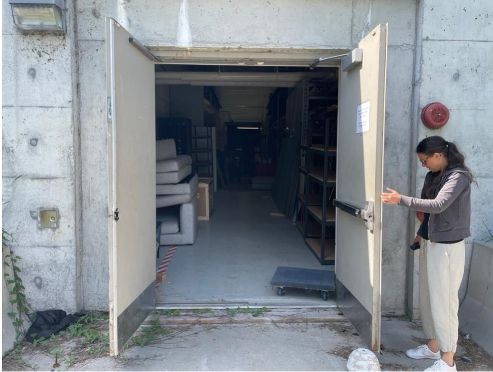
Exterior door, Access 1 - Chemin Macdonald 165 cm (L) 225* cm (H)
