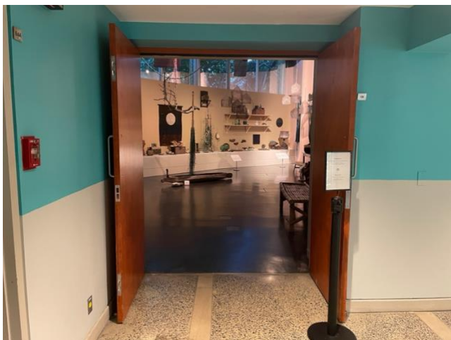
Room 5 entrance and exit door 171,7 (L) x 221,4(H) cm
