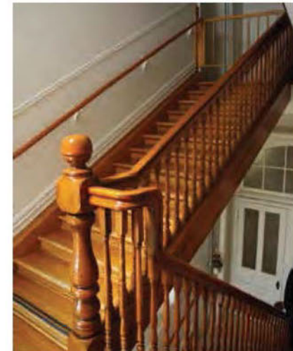
Escalier aile A (Source : Patri-Arch, 2016)
