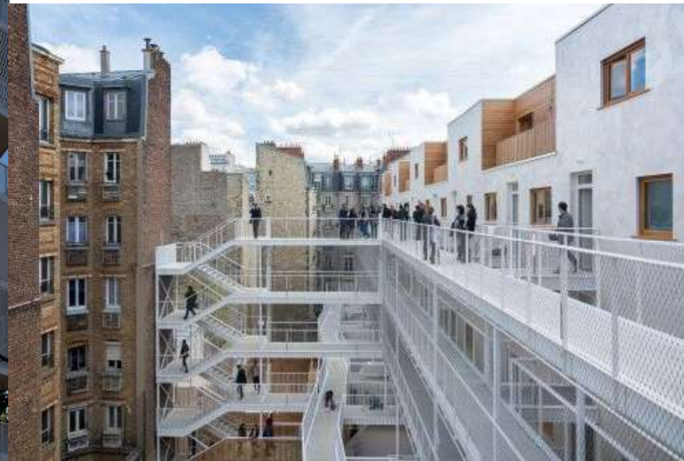
Immeuble Less - AAVP architecture
