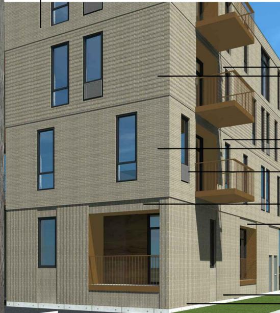
APPAREILLAGE EN PANNERESSES, OU A DEMI-BRIQUE, AVEC UNE RANGEE SUR DEUX EN RETRAIT
