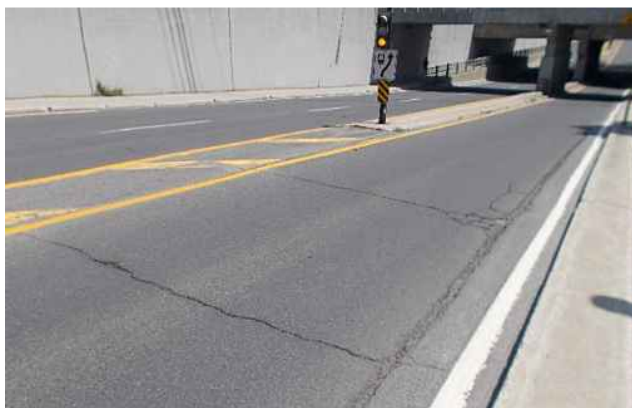
Fissuration transversale et joint froid
