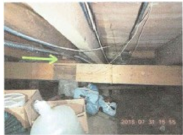
Solive mal supporté.
