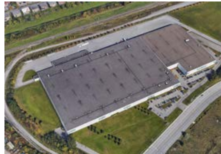
Fig. 73. Centre de distribution Reitmans (Source: Google Street View, 2019)
