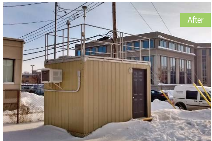
Replacement of the Décarie Interchange station (28)
