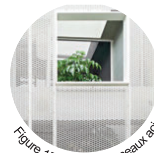
Figure 16 : façade panneaux acier 2
