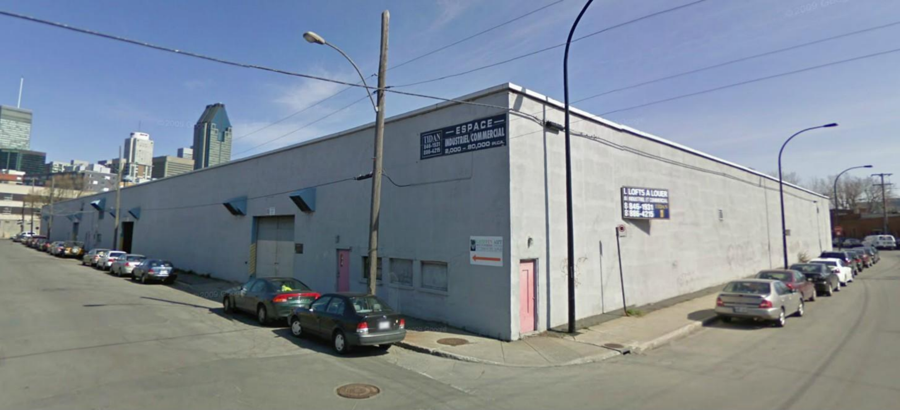
PHOTO SITE NO.2
