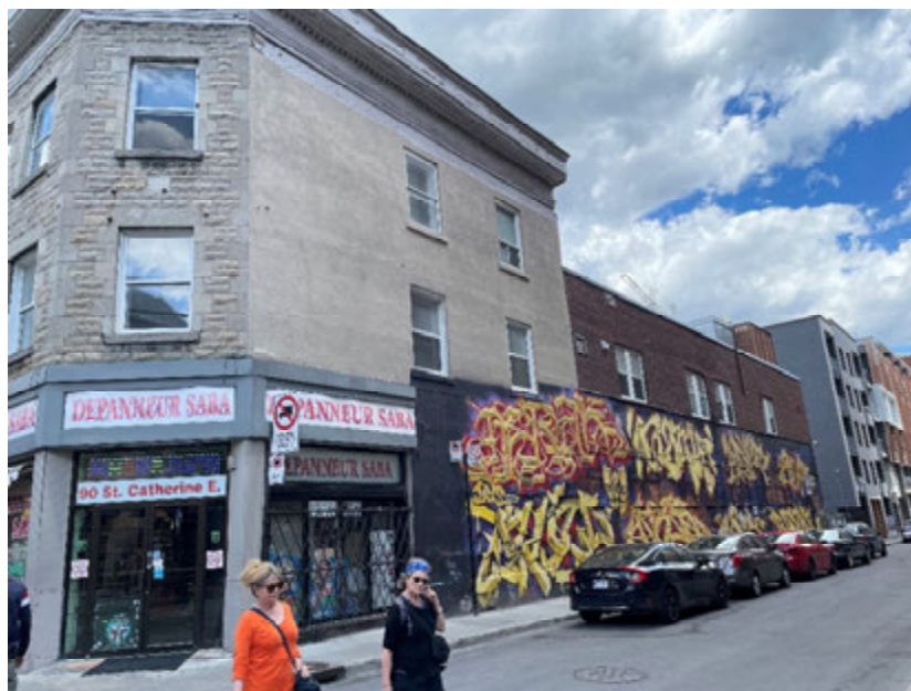
Figure 6 - Façade rue Berger
