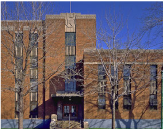
Sandra Cohen and Colin Rose, Kraft Phoenix Cheese Building Montréal. (s.d.), Photographie.
