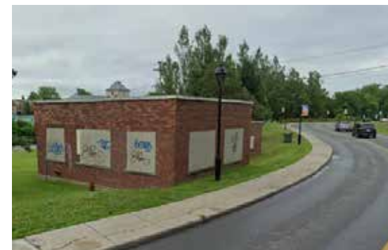
106. Station de pompage
