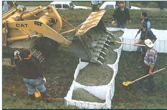
Figure 5: filling operation
