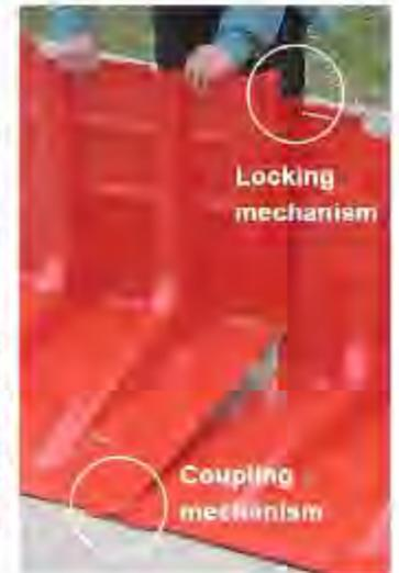
In February 2017 a modification of the locking mechanism was introduced, to facilitate assembly and disassembly. At the same time the height of the pin was somewhat increased. Boxes of newer and older type still fit together, but because of the increased height of the pin new boxes should be put to the left, and old ones to the right, to facilitate dismantling.
