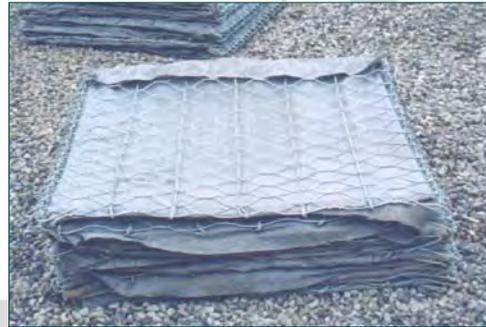
Figure 7: clean, fold and repack the unit for next use
