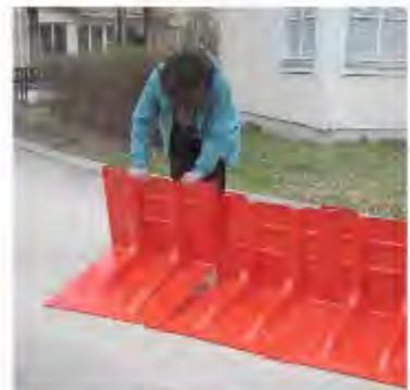
The boxes are easy to handle and move, and you can also adjust the setting of a constructed boxwall as long as the water has not started to press firmly against the base. But you must avoid dragging the boxes on the ground, as the sealing strips on the underside are vulnerable to wear.
