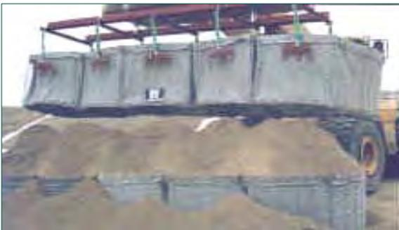
Figure 6: FLEXMAC® DT unit lifting operation
