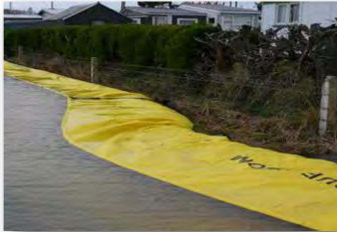
Picture 10 - Water-Gate Simulation Protection - 604 m on Havenweg
