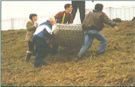
Figure 4: manual transportation of FLEXMAC® DT unit
