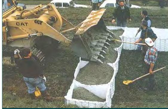
Figure 5: filling operation
