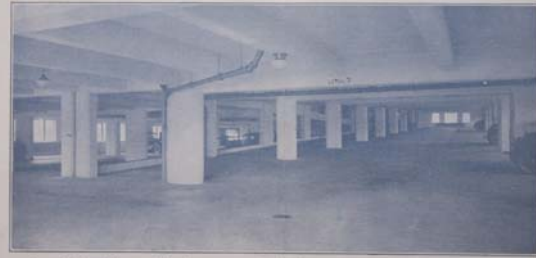
One of the Floors. All above ground, having natural light and ventilation on four sides.
