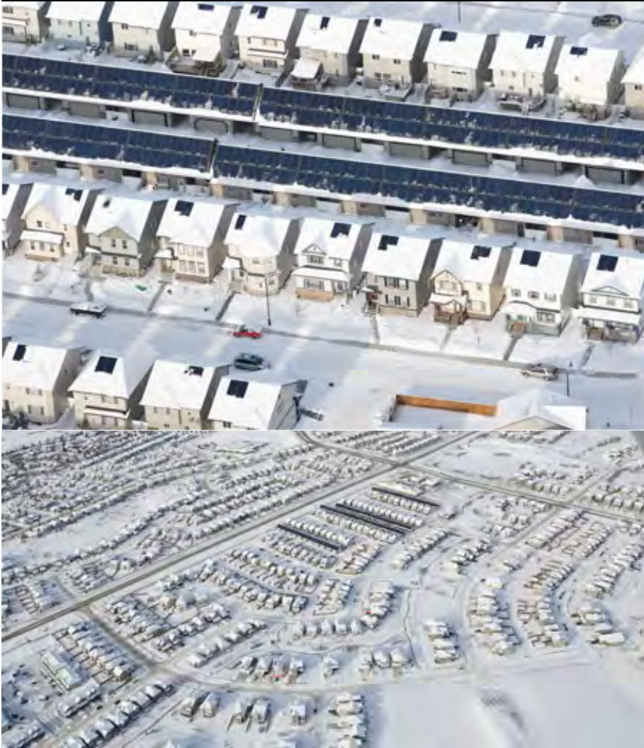
Drake Landing Solar Community, Alberta
