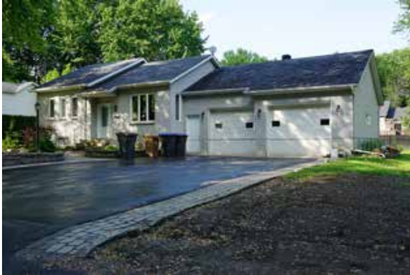
Above: A high water mark is visible across the garage doors and around the side of the house.
