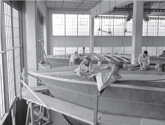
«Workers covering the hulls of motor torpedo boats under construction at Canadian Power Boat Company with linen fabric, Montreal, Québec, Canada, 24 April 1941.» (Credit: Canada. Dept. of National Defence / Library and Archives Canada / PA-132179)
