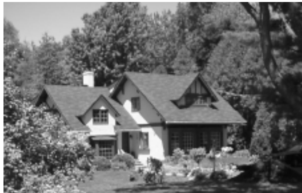
2.U.4 Le 23, avenue Tunstall
