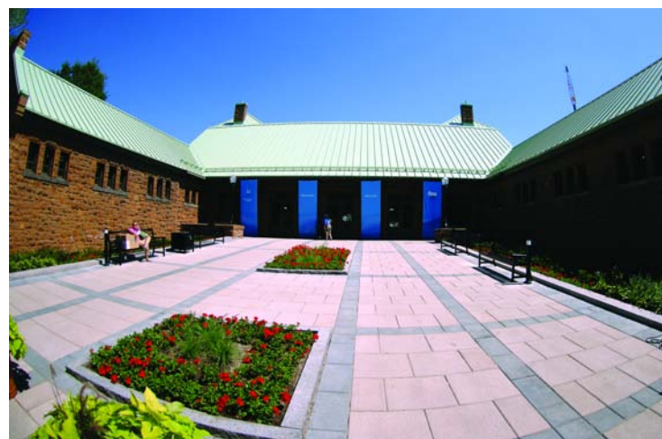
Fully restored, the Baigneurs pavilion recovered its lustre of yesteryear.
