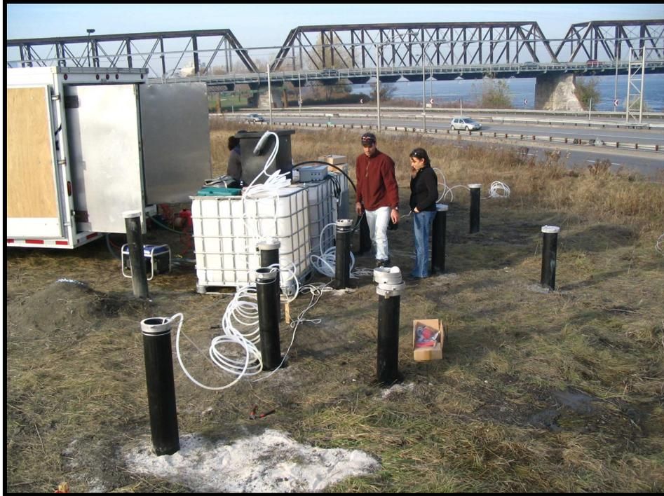
PHOTO 9 : VUE DES INSTALLATIONS POUR LE PROCESSUS DE TRAITEMENT DE LA ZONE RÉACTIVE IN SITU
