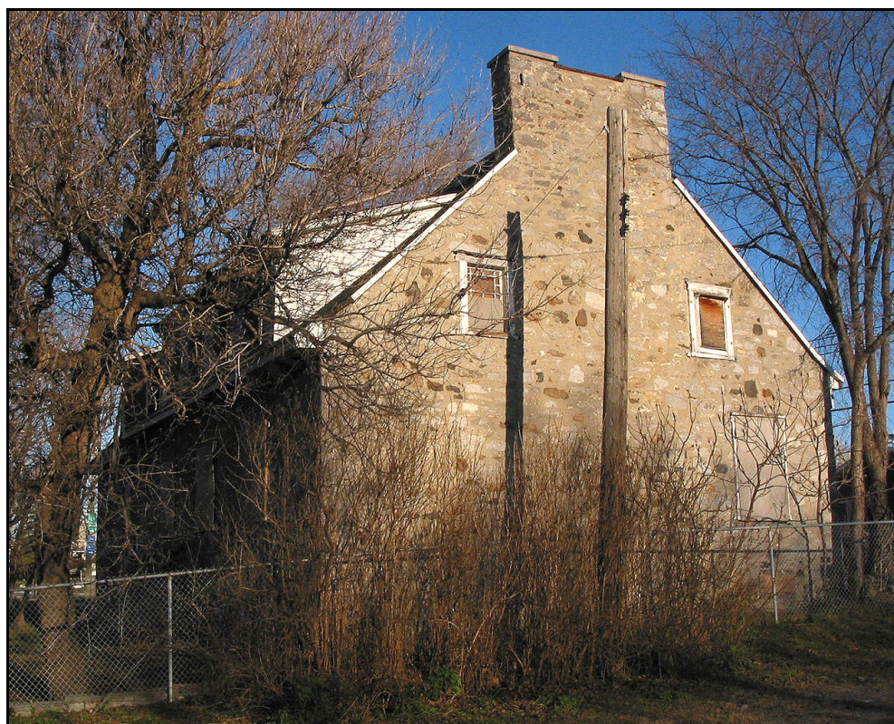
Figure 2.4. Façade ouest, 4251, boulevard Gouin Est, 2006
