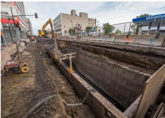
Construction of a watermain by trenching. This method requires the excavation of a portion of the street in order to dig a trench to install the watermain. Once the work is completed, the street is rebuilt.
