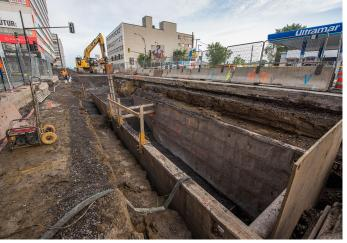
Construction of a water main in trenches. This method requires excavation of part of the street to dig a trench where the main will be installed. After the work is complete, the street is rebuilt.
