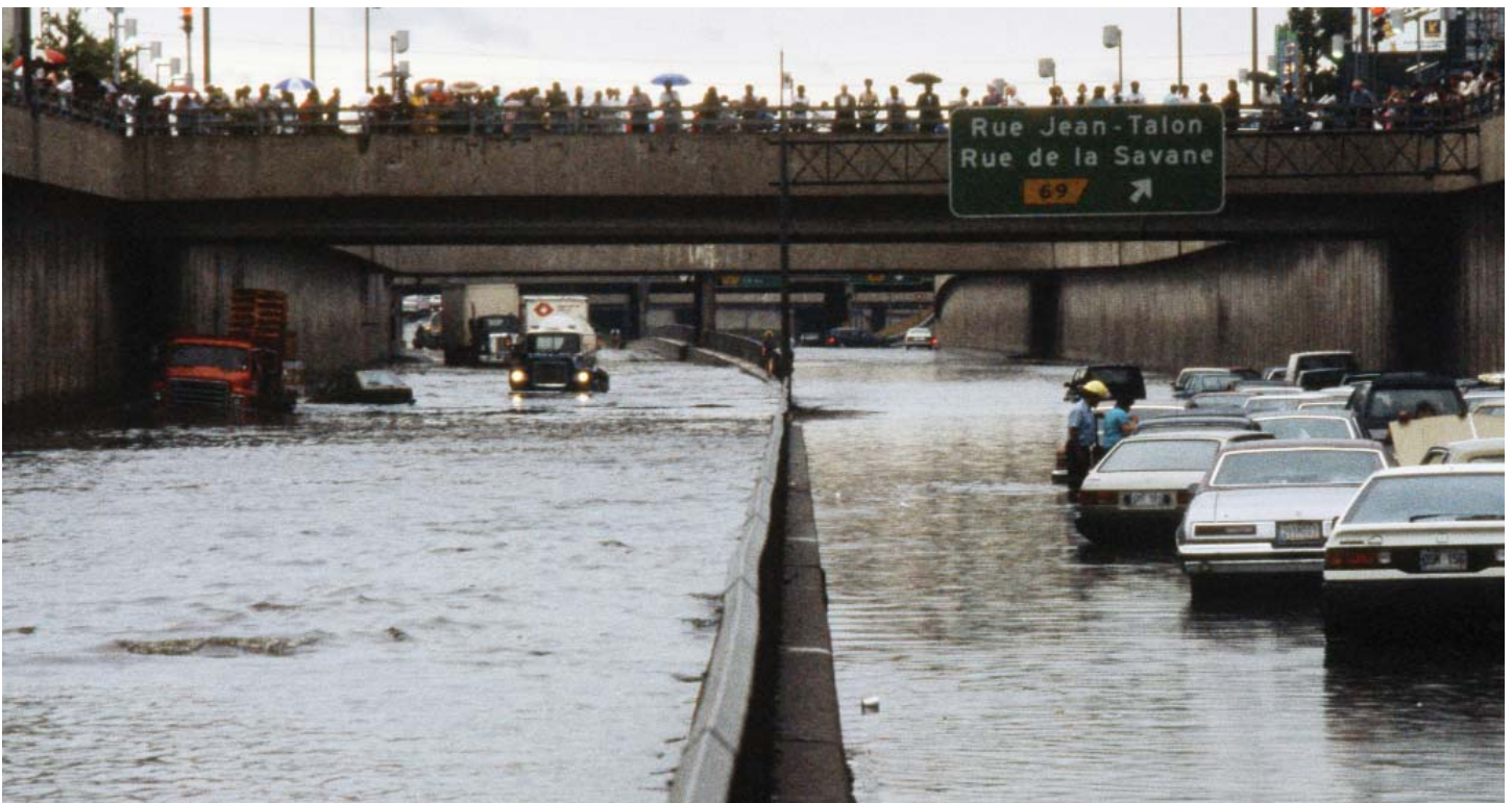
On July 14, 1987, Décarie Expressway looked like some rapids after a rainfall of 101.2 mm in just two hours. Credit: © La Presse
