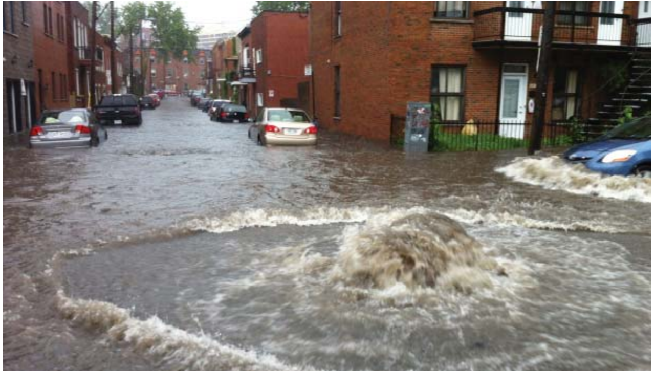
Sewer system overflow following intense rainfall in Montréal on May 19, 2012 Credit: © Métro newspaper, www.journalmetro.com
