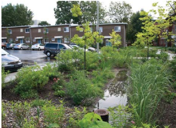
Bioretention basis at the Habitations Jeanne-Mance parking lot in Ville-Marie
