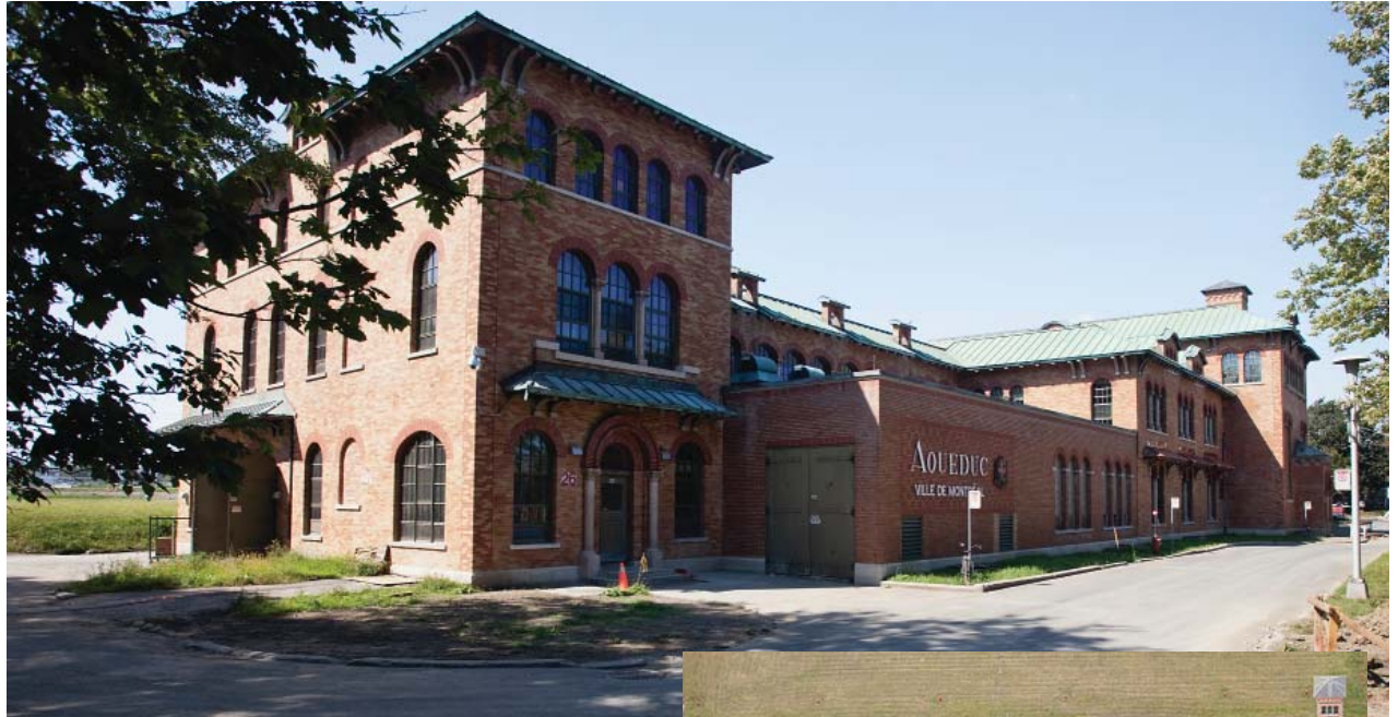
Atwater Drinking Water Production Plant
