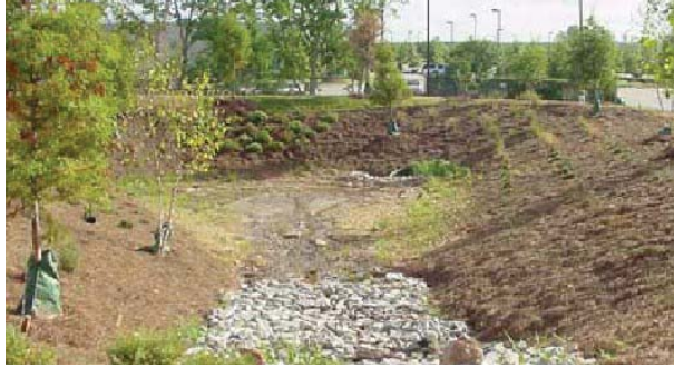
Dry retention basin at the train station between Saint-Léonard and Montréal-Nord
