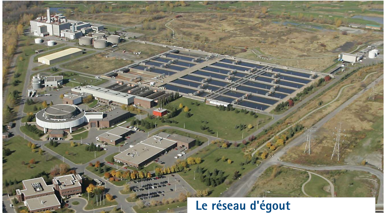
Jean-R. Marcotte Wastewater Treatment Plant
