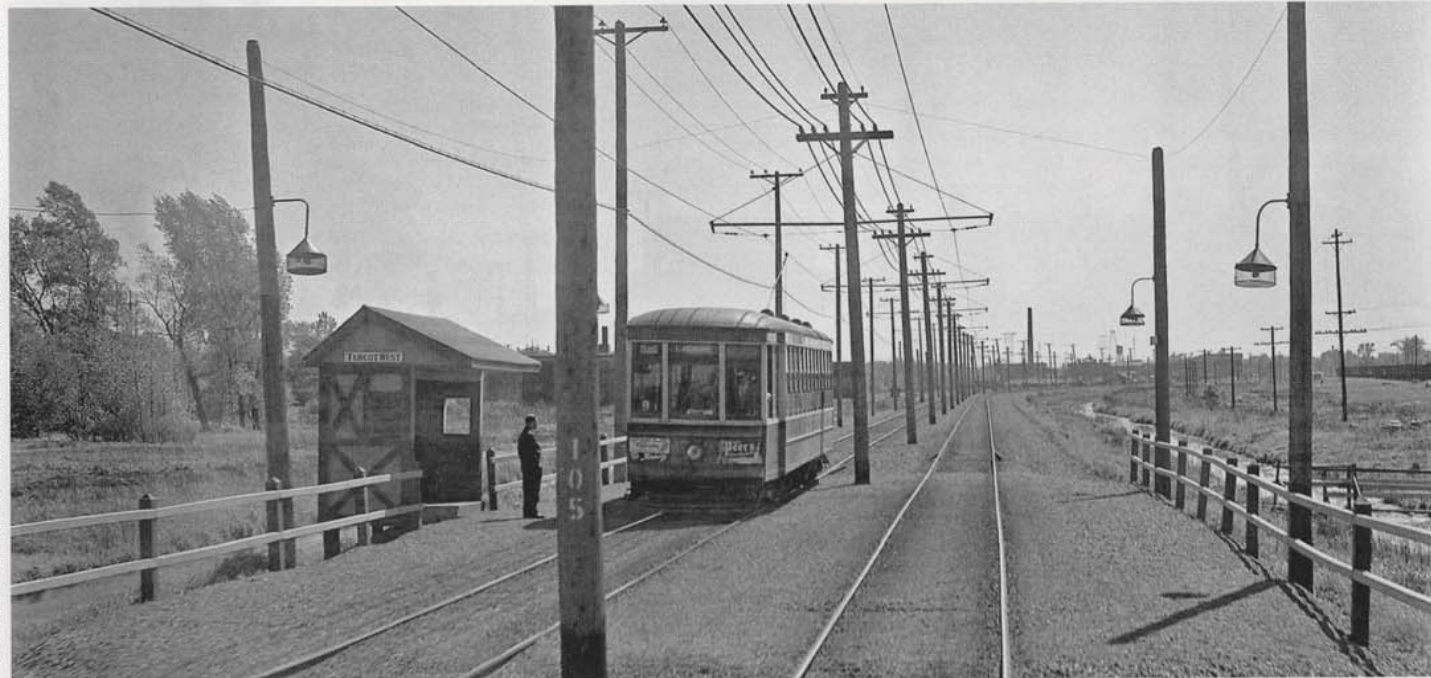
This is a view of eastbound 1550-series car stopped for passengers at Turcot West station when enroute to Place d'Armes. (Author's Collection)
