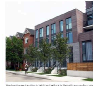
New townhouses transition in height and setback to fit-in with surrounding context.
