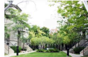
Sufficient separation distance allows for attractive landscaping between buildings, good access to sunlight and sky views. Avoid more than 3-5 steps up or 8-9 steps down to the units to further improve the shared spaces between buildings.
