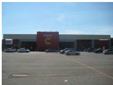
Oversized parking lots and absence of green islands, intersections on boulevards des Sources and de Pierrefonds
