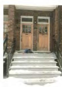
BALCON ET MARCHES D'ENTRÉE À REMPLACER (VÉRIFIER ÉTAT DE LA STRUCTURE). REVÊTEMENT DE PLANCHER ET MARCHES EN BOIS/COMPOSITE FIBERON OU ÉQUIVALENT. GARDE-CORPS À REMPLACER PAR ALUMINIUM SOUDÉ NOIR
