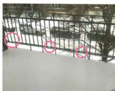
GARDE-CORPS EXISTANT EN MÉTAL ROUILLÉ PERCÉ DANGEREUX, REMPLACER PAR MÊME MODÈLE RÉGLEMENTAIRE 42" EN ALUMINIUM SOUDÉ NOIR (BARROTINS À 4" c/c).
