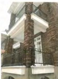
BALCONS À REPARER À L'IDENTIQUE AVEC REVÊTEMENT DE PLANCHER PIN EMBOUTI VÉTÉ TEL QU'EXISTANT GARDE-CORPS MÊME MODÈLE EN ALUMINIUM SOUDÉ NOIR
