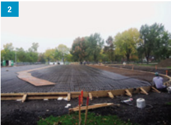
Installation of the refrigeration system.
