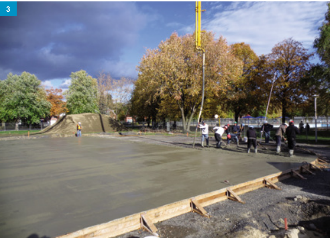
Pouring of the concrete slab.
